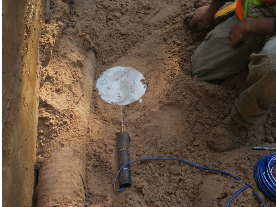
Figure 109. Installation of vertical EPC at drain tile at Schwartz Road Bridge
