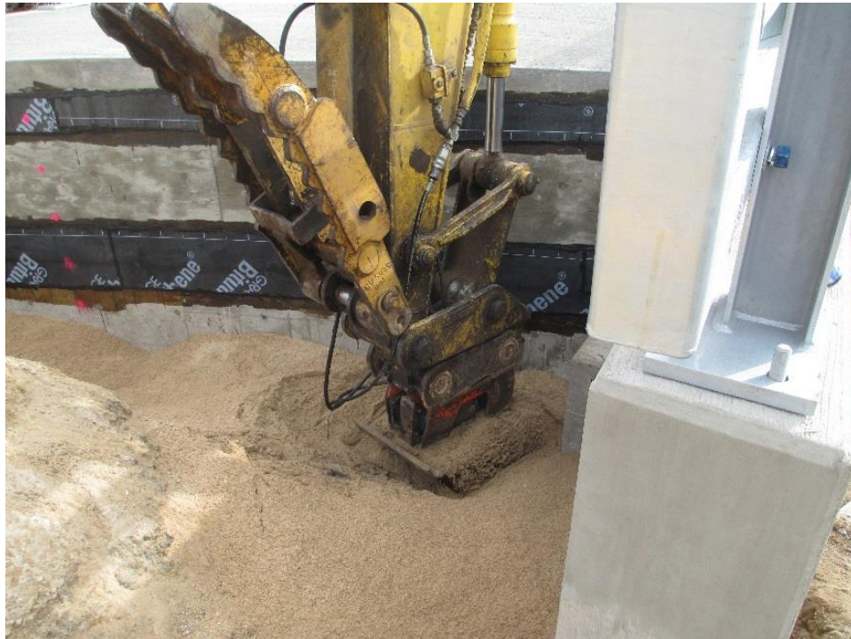
Figure 133. Compaction with vibratory compactor attached to an excavator
