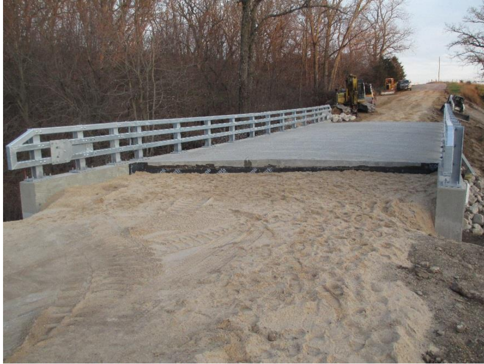
Figure 134. Badger Road Bridge after backfilling abutment
