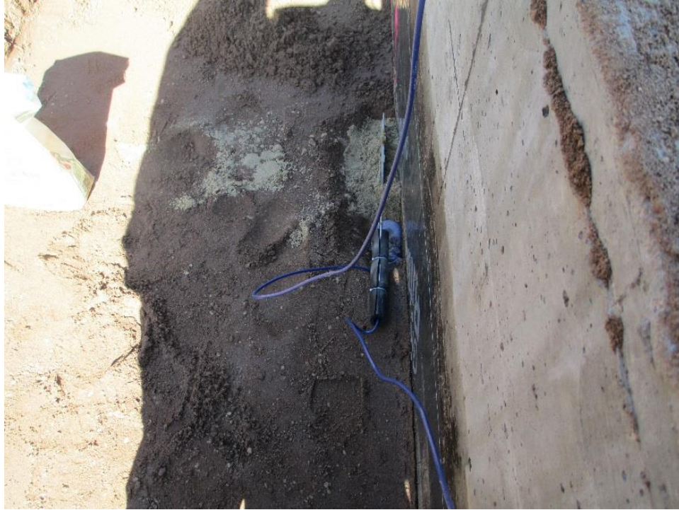
Figure 126. Lateral EPC installation at Hobbles Creek Bridge
