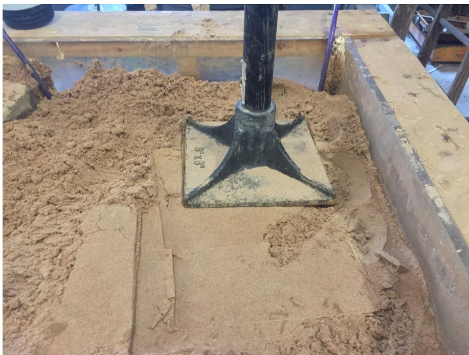
Figure 31. Compaction of fill material using a hand tamper
