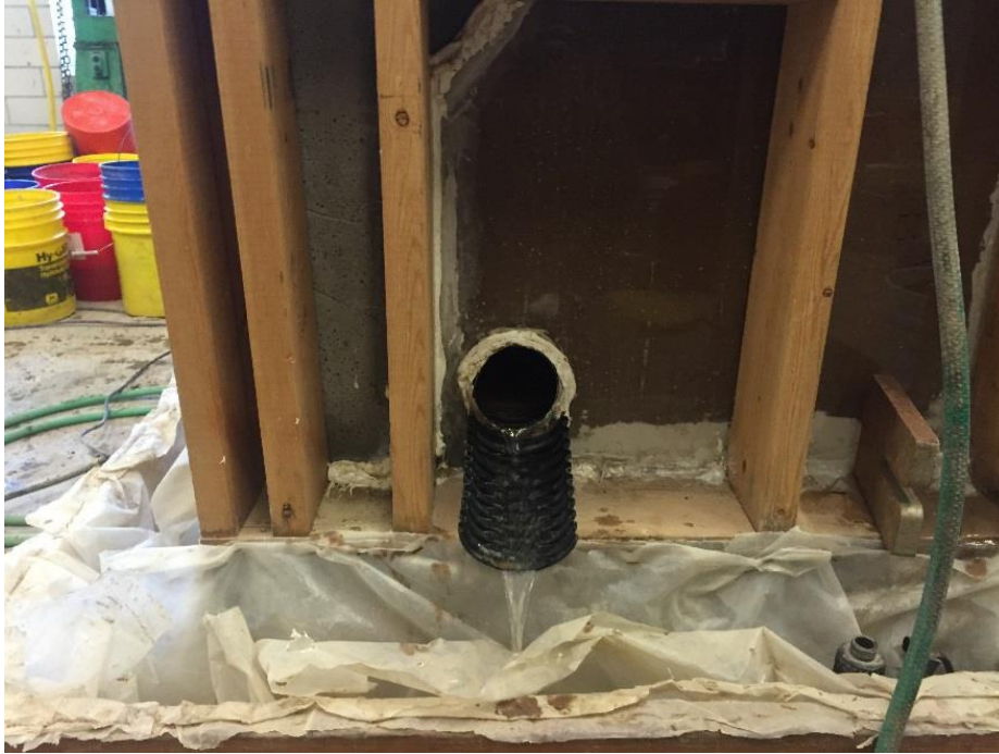
Figure 34. Water draining through the drain tile during dissipation test
