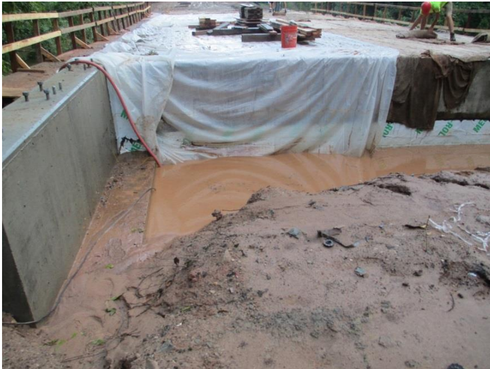
Figure 100. Poned water in the abutment excavation at Schwartz Road Bridge
