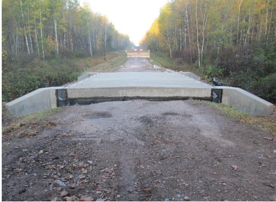
Figure 116. Hobbles Creek Bridge west abutment before backfilling
