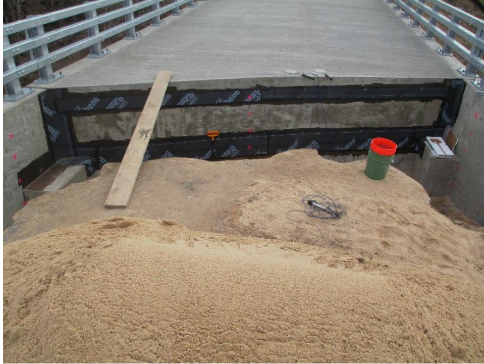
Figure 132. Badger Road Bridge before backfilling on west abutment
