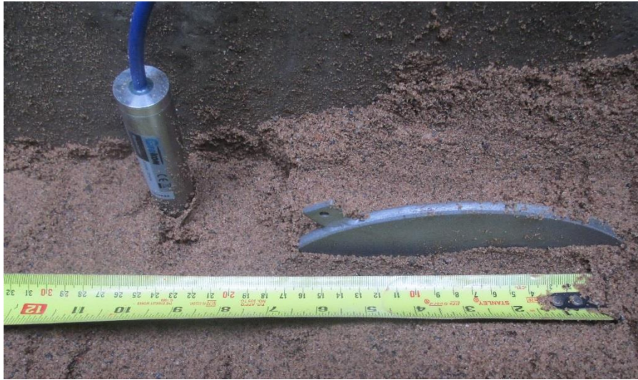
Figure 87. Photograph of an installed PP (left) and EPC (right) sensors
