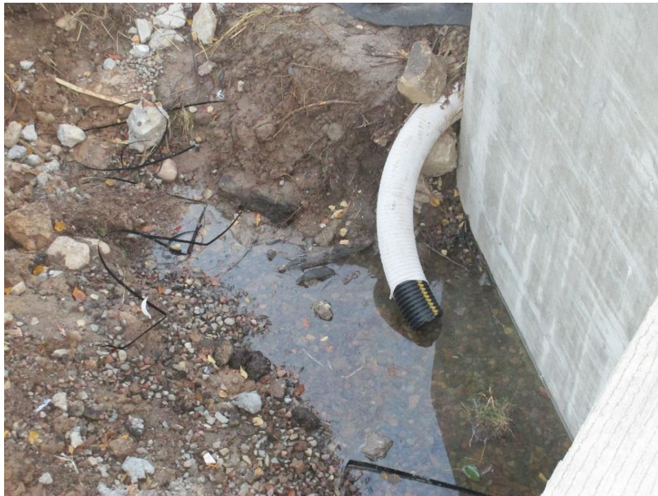
Figure 117. West abutment excavation at Hobbles Creek with standing water
