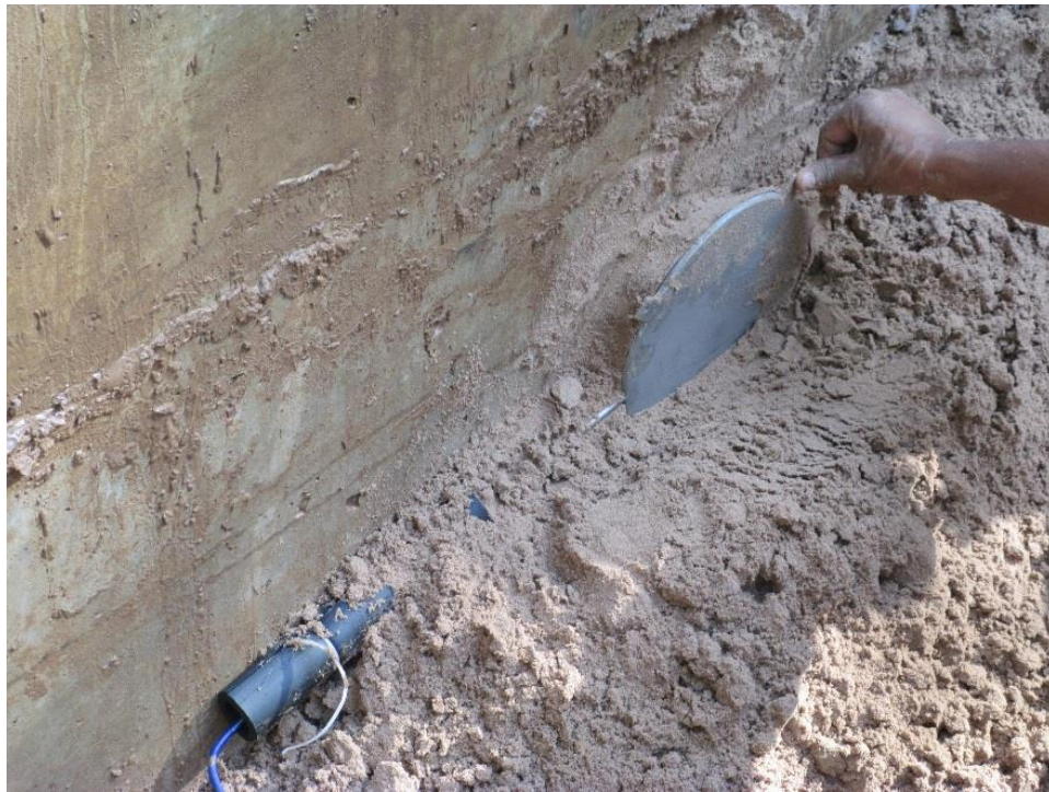
Figure 108. Installation of lateral EPC at drain tile at Schwartz Road Bridge
