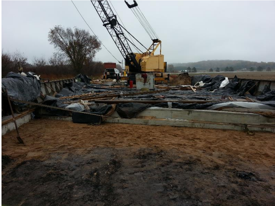
Figure 81. Slovak Valley Creek Bridge west abutment near its final elevation
