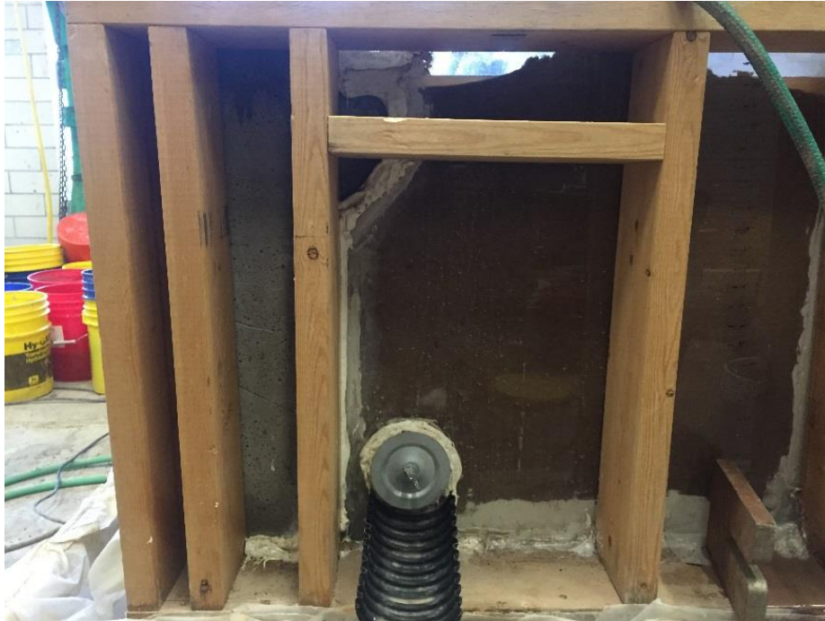
Figure 33. Drain tile plugged for saturation
