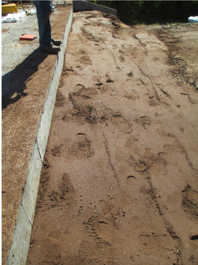
Figure 118. Hobbles Creek Bridge after backfilling
