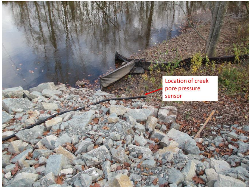
Figure 110. Location of creek pore pressure sensor at Schwartz Road Bridge
