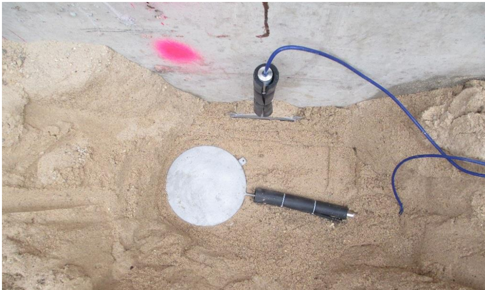
Figure 140. Sensor installation behind Badger Road Bridge
