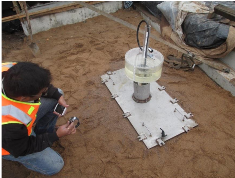
Figure 37. Corehole permeability test setup
